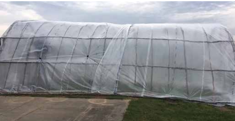
Photos: (Clockwise) The unique hoop house built as part of a Sokaogon Chippewa Community agriculture project. Tribal youth volunteers learn hoop house construction during a Sokaogon Chippewa Community agriculture project. Black spruce, like the tree shown below developing pine cones, were grown from seedlings and planted on reservation lands.
