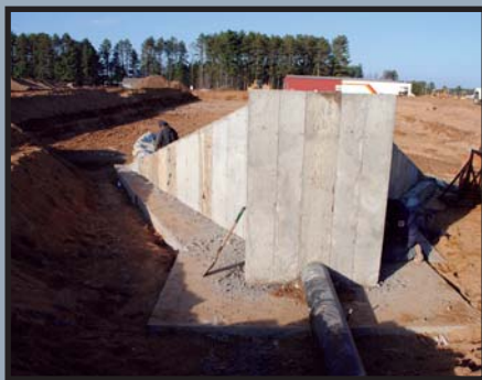
Construction of the outlet structure for the facility
