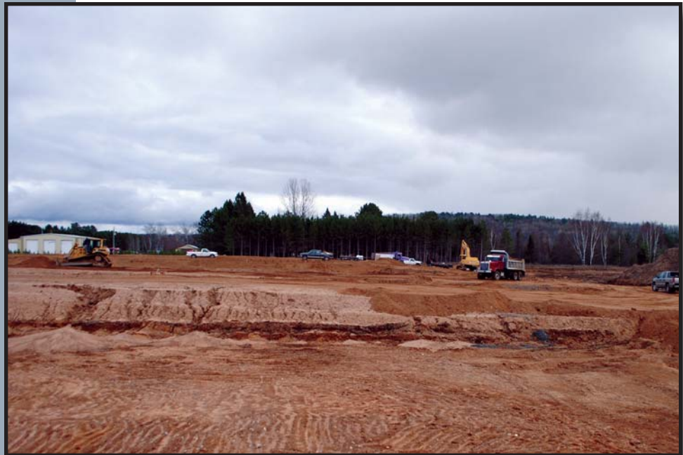
Construction beginning on the Mole Lake aquaculture facility
